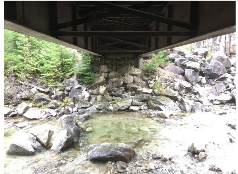
Right Bank Abutment when facing downstream
