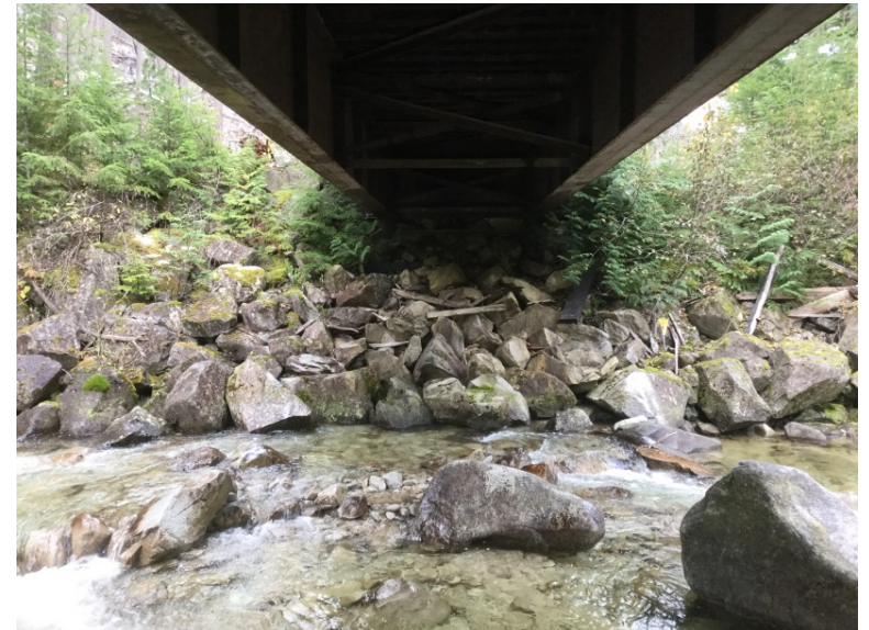
Left Bank Abutment when facing downstream
